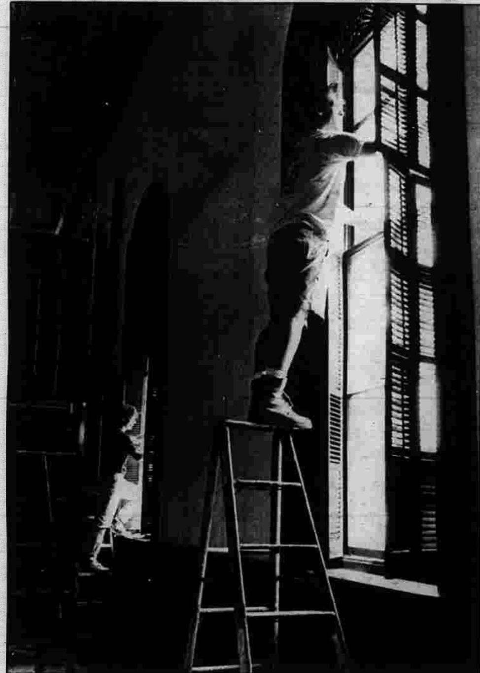
WINDOW WORK — A pair of workers puts finishing touches on the hall auditorium windows recently.
